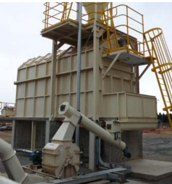
Storage bin with screw conveyor to hammermill.
